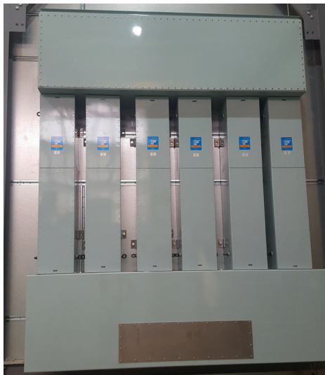
Array of EMP protection filters installed on an EMP shield
